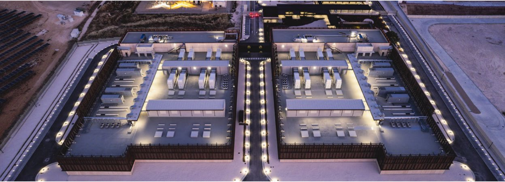
Data Processing Centre, built by FCC Industrial, in Torija (Guadalajara).
