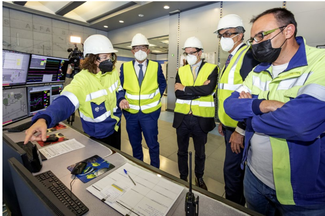
During the conference, the factory management presented its Energy Transition and Climate Neutrality Plan 2021-2030.
